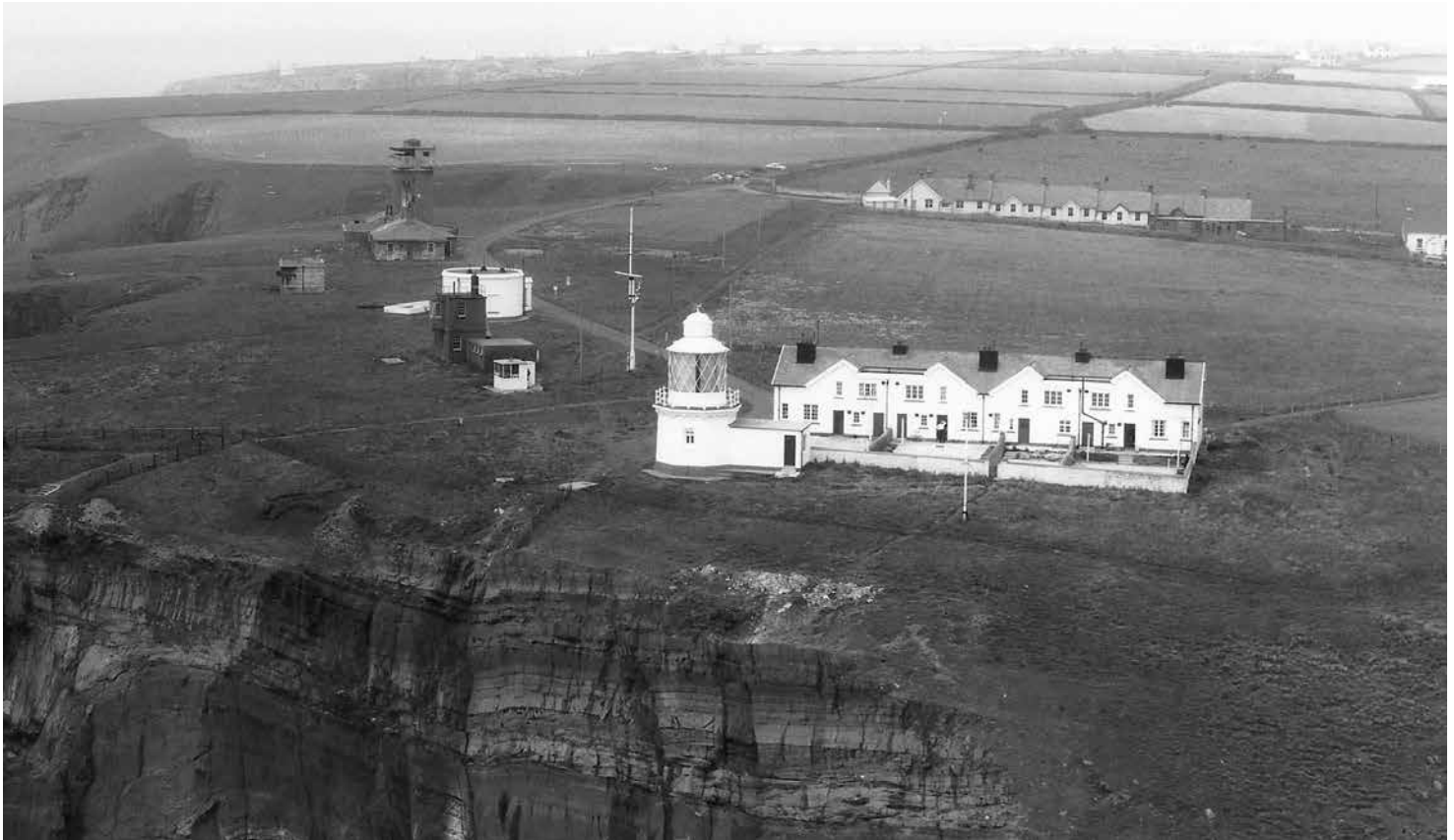
ABOVE: An aerial view of the present lighthouse station at St. Ann's Head near Milford Haven in Pembrokeshire. Like South Foreland, it was once a two-light station, the original High light almost invisible here in the left centre. It was discontinued in 1910. The low light was shown from the 1844 tower in the centre and remains in use today. The lighthouse cottages have been significantly altered since the nineteenth century.
